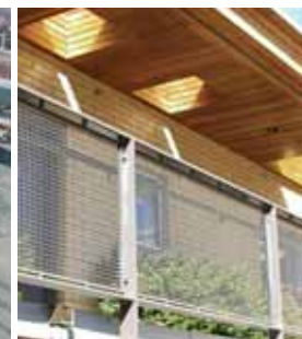
etched glass and applied visual markers including simple dot patterns deter bird strikes
