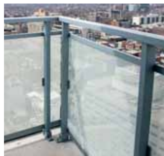
etched glass and applied visual markers including simple dot patterns deter bird strikes
