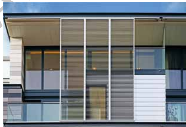
fenestration patterns and window shading can increase bird safety
