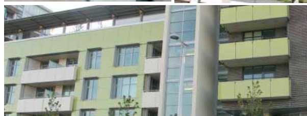
sample strategies to increase reflectivity and reduce the appearance of clear passage through balconies
