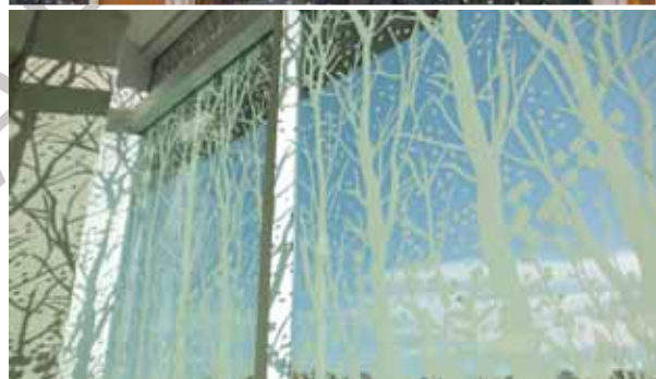
etched glass and applied visual markers including simple dot patterns deter bird strikes
